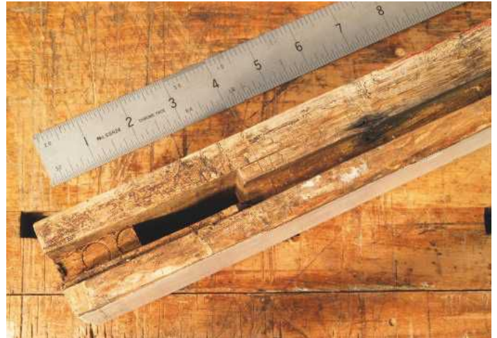
▲ Pic.2 Close up of the original mortise
